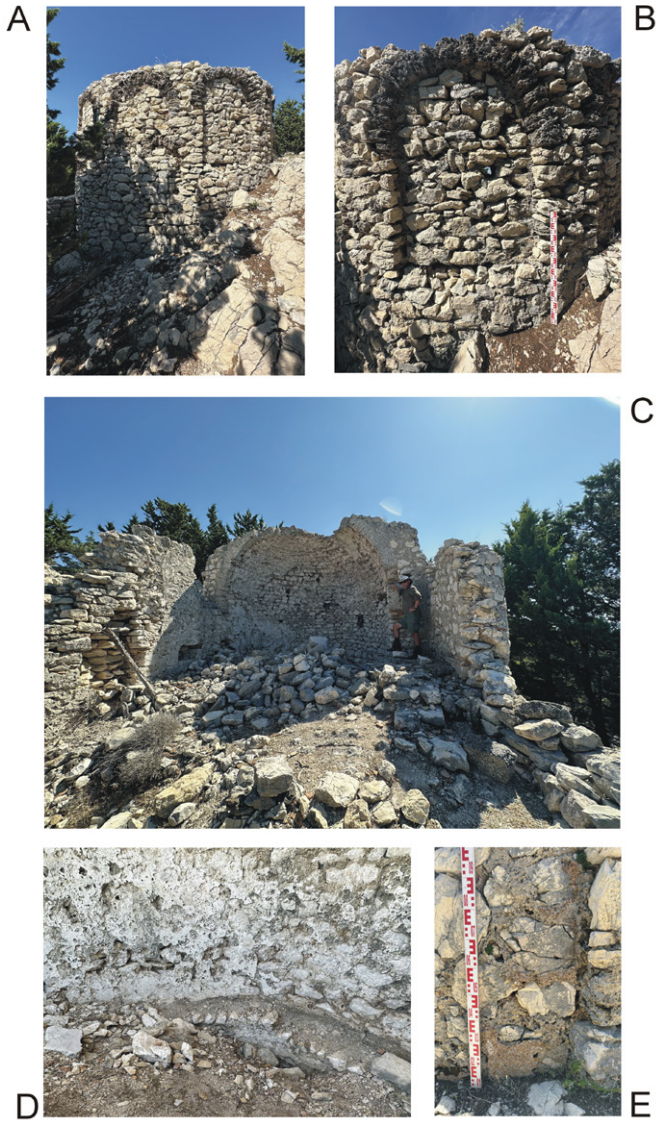
Fig. 11. A: Apse of the early Byzantine church preserved inside the fortress in Barbat (Photo: F. Welc). B: The niche of the apse. Its upper arch was made of travertine (Photo: F. Welc). C: View of the interior of the church's apse (Photo: A. Konestra). D: View of the bench preserved in the interior of the apse (Photo: F. Welc). E: Lower external wall of the apse covered with waterproof plaster (Photo: F. Welc)
