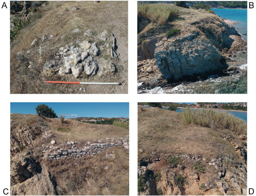
Fig. 3. Preserved relics of late antique walls on Lukovac Island. A. Remains of a buttress in the south-western part of the island. B. Remains of a long buttress in the north-eastern part of the island. C. The outer wall of a cistern. D. Relics of the perimeter wall with the remains of a buttress preserved in the south-eastern part of Lukovac Island. Photos: F. Welc
