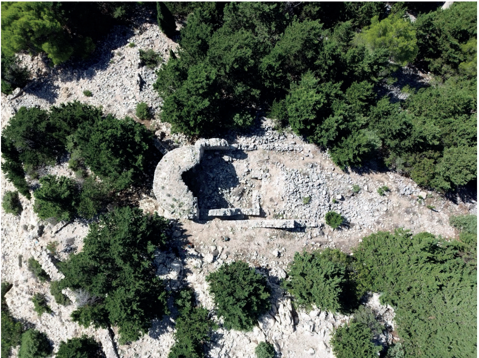
Fig. 10. Top: aerial view of the Byzantine fortress preserved in the Barbat area (St. Kuzma and Damjan), southern part of the island of Rab. Photo: F. Welc. Bottom: aerial view of the remains of an early Byzantine church. In the foreground, the perfectly preserved ceiling of the apse. Photo: F. Welc
